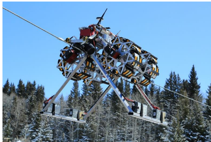
Bird markers being installed by a drone operated robot.
