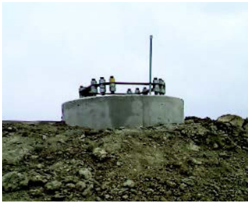
Above: AltaLink will excavate and install transmission structure foundations.
