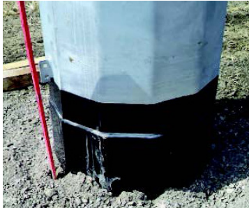
Above: Structure bases are then attached to the foundations.
