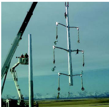
Above: AltaLink will assemble and erect steel pole structures.
