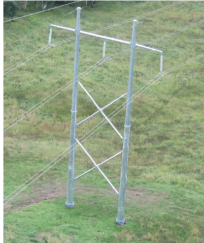
The existing steel lattice structures are in the picture to the left. The new steel H-Frame structures will look similar to the picture on the right.
