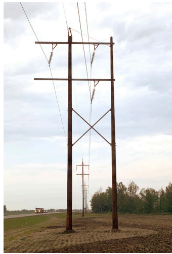
The H-frame structures will look similar to the photo above.
