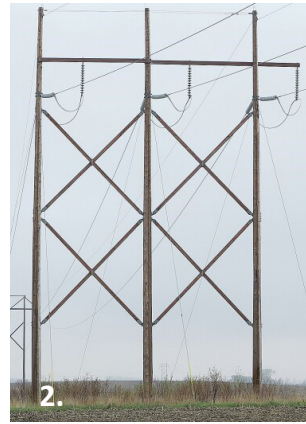
1. Sample proposed monopole structure on 1002AL. 2. Sample proposed three-pole structure on 1002AL. 3. Sample proposed monopole structure on 1002L.
