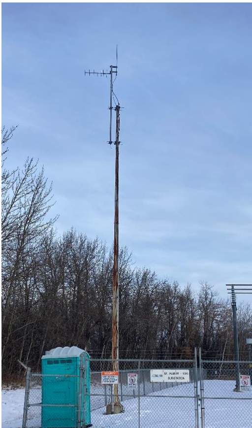
The new telecommunications pole will look similar to the photo above, but will be steel.
