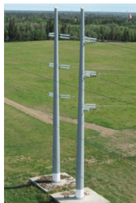
Left: an example of the proposed monopole structures that will be used to connect EPCOR's proposed transmission line.
