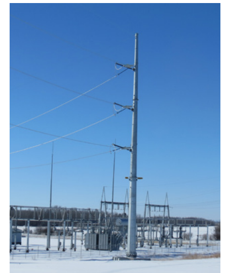
The steel double-circuit lattice structure on the 920/921L (above) will be replaced with two new single-circuit monopoles made of steel (below).
