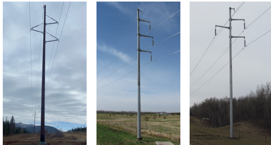
Above: Steel single monopole structures will be used throughout the new transmission lines. These monopoles will be between 25 to 32 metres tall.
