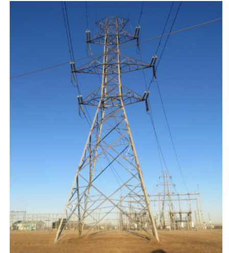
The steel double-circuit lattice structure on the 920/921L (above) will be replaced with two new single-circuit monopoles made of steel (below).
