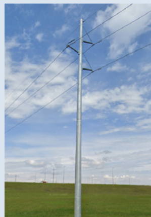
For the proposed 1047AL transmission line, the monopole structures will look similar to the photo above.
