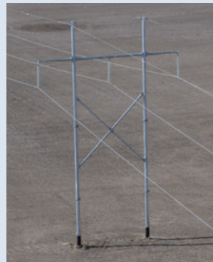
For the proposed 1047AL transmission line, the H-frame structures will look similar to the photo above.
