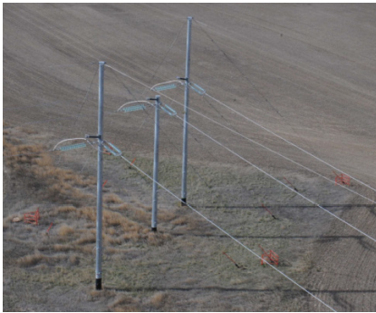
Above: Sample three pole dead-end structure
