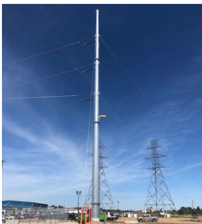
Above: Sample monopole dead-end structure
