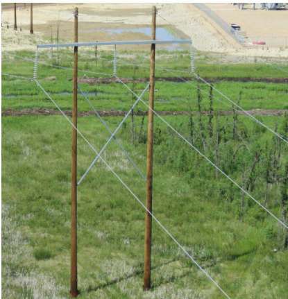
Above: Sample H-frame structure
