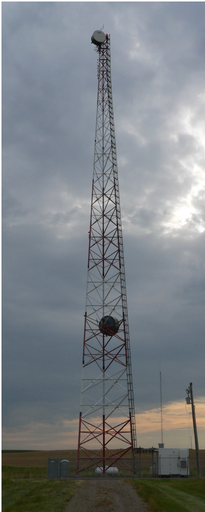
Top photo: The structures required for the new short 138 kV lines will look similar to the above.
