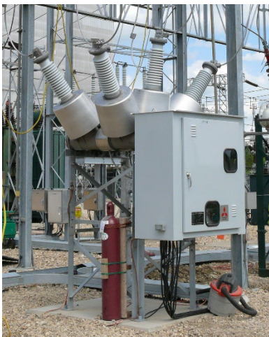
The 69 kV circuit breaker looks similar to the picture on the left. The 240 kV circuit breakers look similar to the picture on the right.
